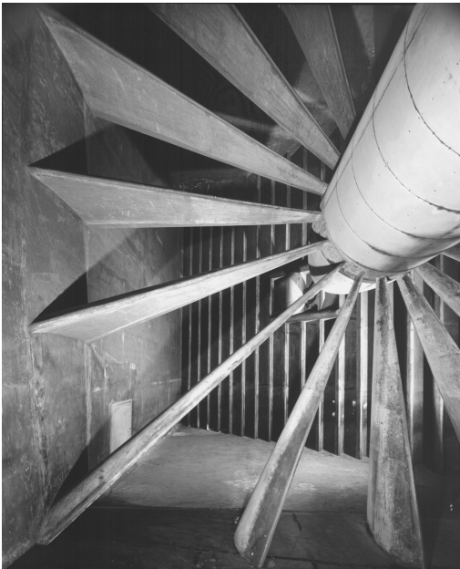
Figure 1 Before the restoration of Q121, taken from inside the wind tunnel, behind the mahogany fan, showing in the foreground the fan shaft supported by aerodynamic concrete blades, with the concrete air-turning veins in the distance. (The Downland Partnership)
