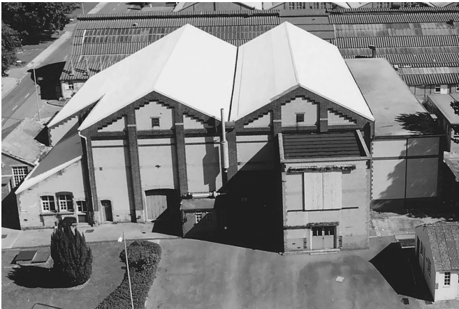
Figure 8a R52 in 1999 showing extensions to the original 1916 wind tunnel building. (Farnborough Air Sciences Trust)
