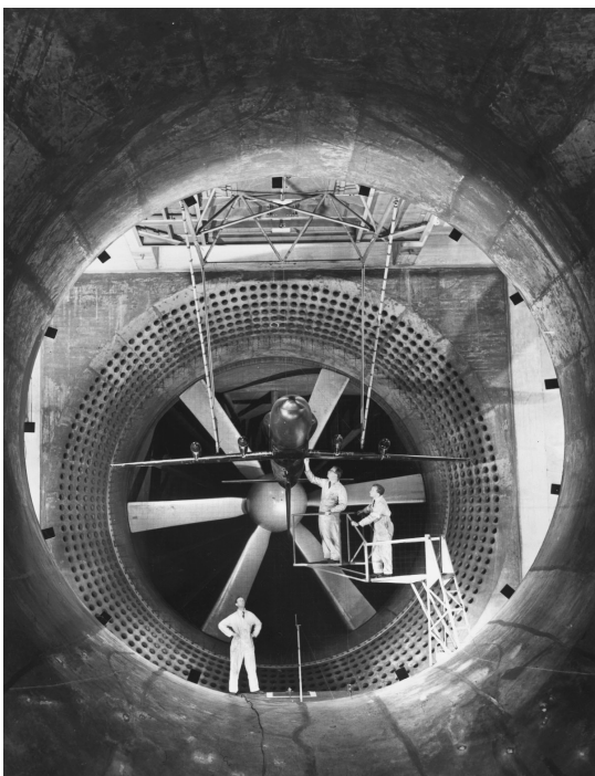
Figure 4 Archive photo of testing in the Q121 wind tunnel. (Farnborough Air Sciences Trust)
