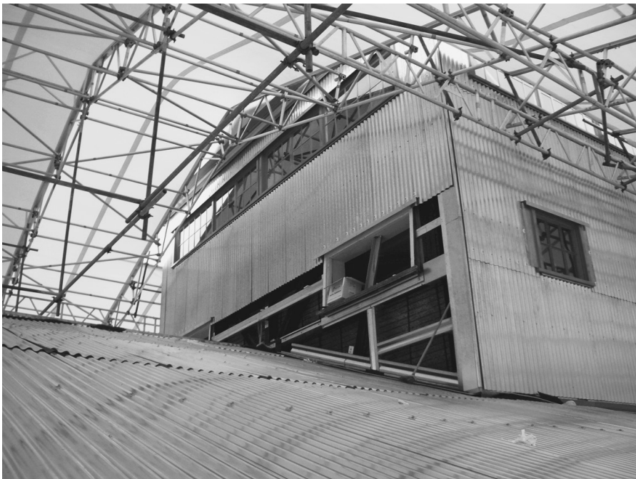
Figure 10 View from the scaffolding looking up to the fourth floor of Q121 during replacement of the original asbestos coated corrugated steel cladding with new corrugated Rheinzink cladding.
