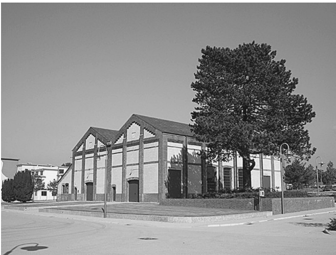
Figure 8b R52 on completion of the repair contract. (Julian Harrap Architects)
